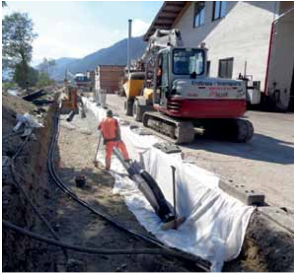
HWS-Mauer in Bau ....
